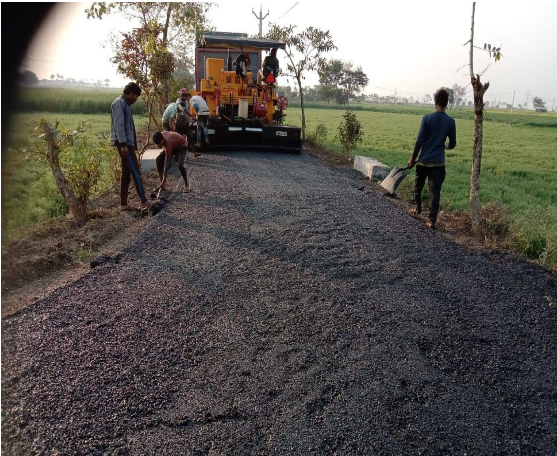
Figure 4.4 Laying of asphalt using paver
