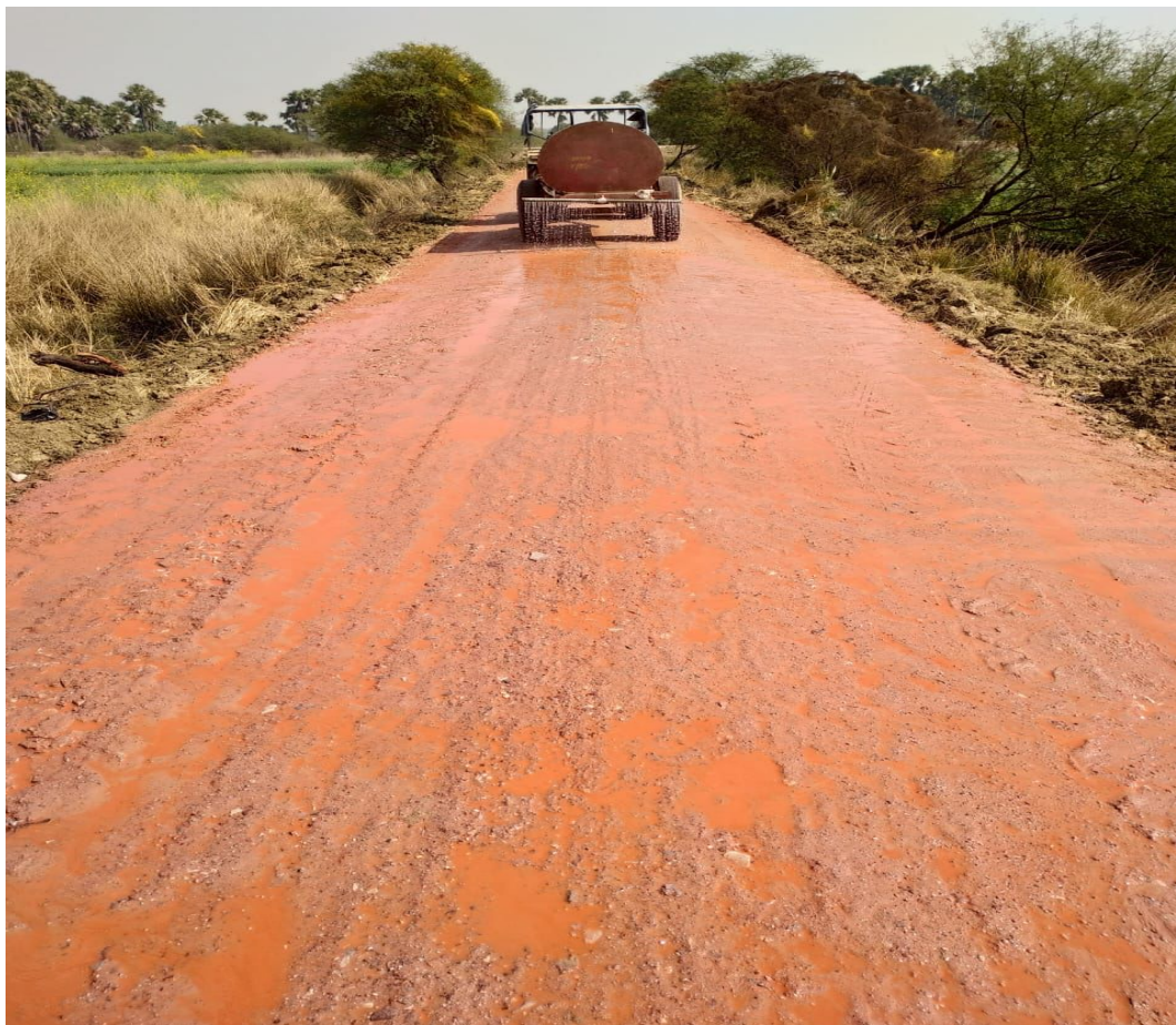
Figure 3.13 Laying of binding material and providing water assistant
