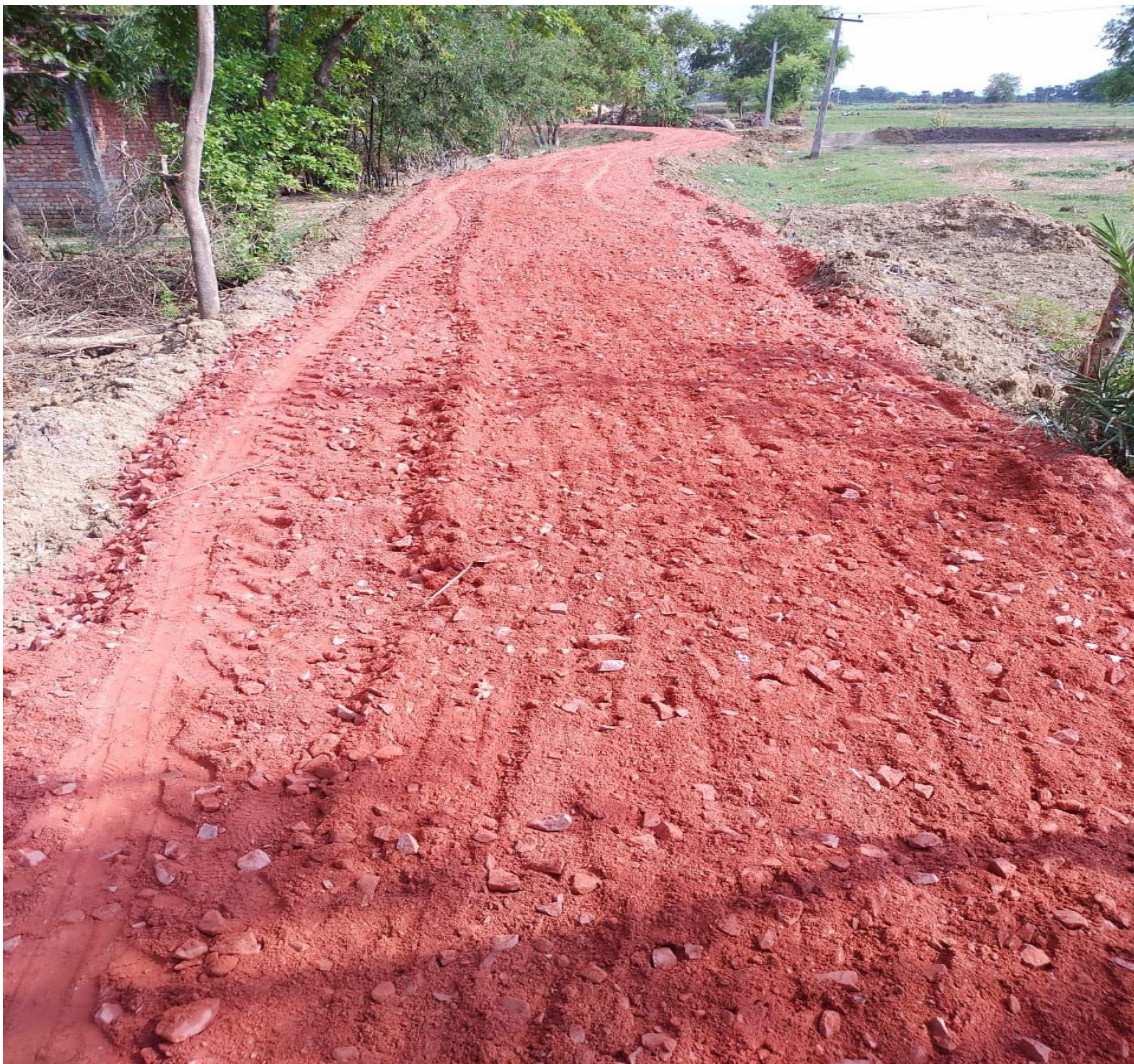
Figure 5.2 Laying of GSB after earthwork
