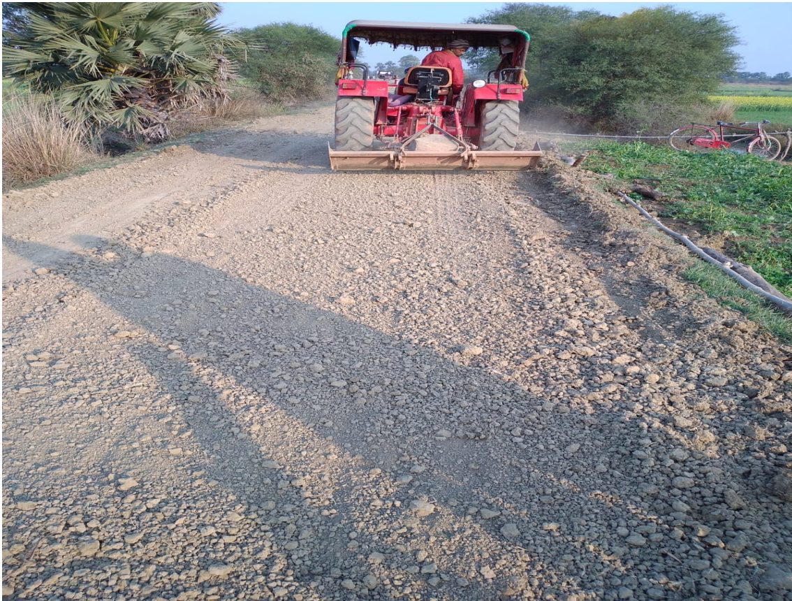
Figure 5.1 Levelling of earthwork using tractor grader
