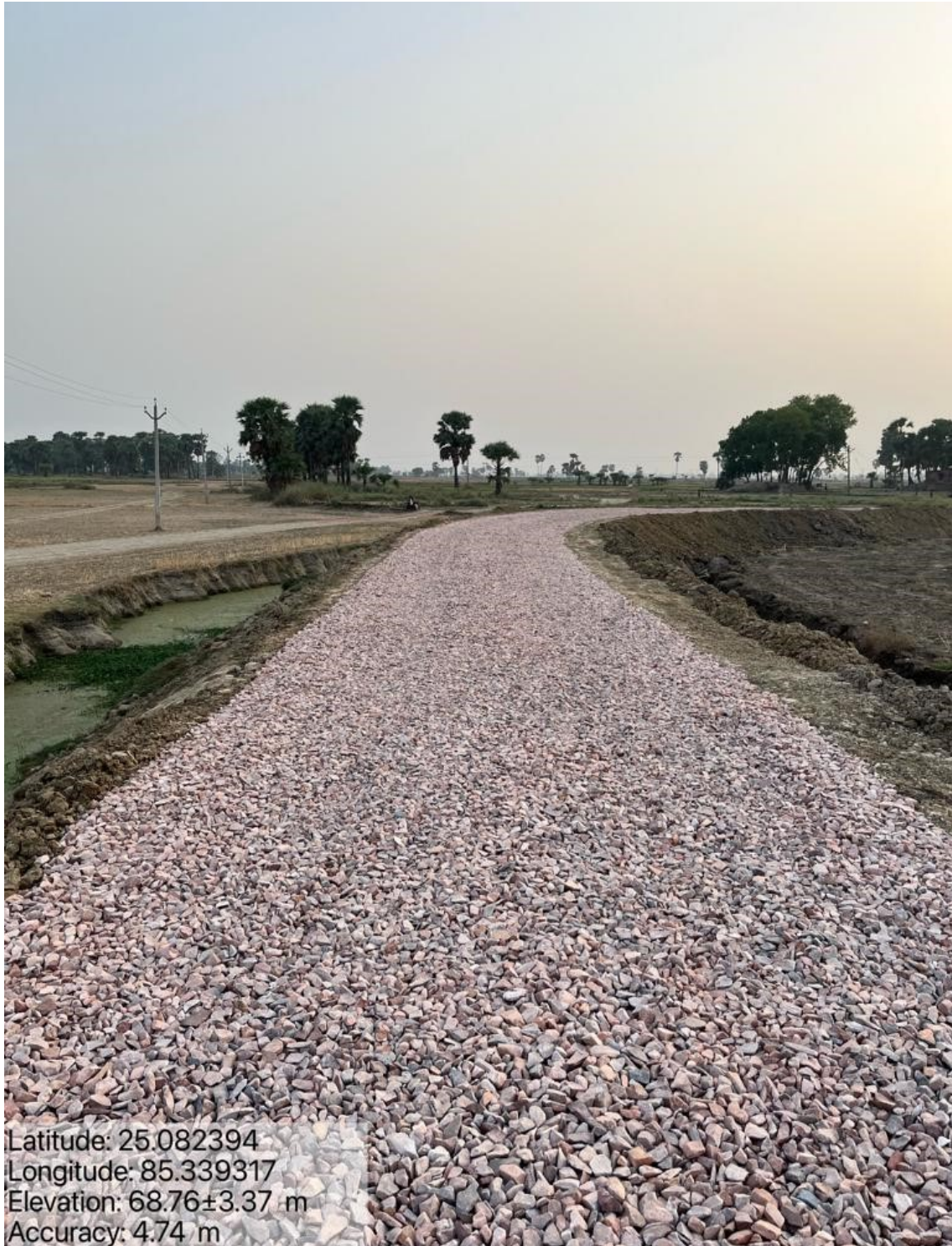
Figure 3.11 WBM/Grade-3 after compaction
