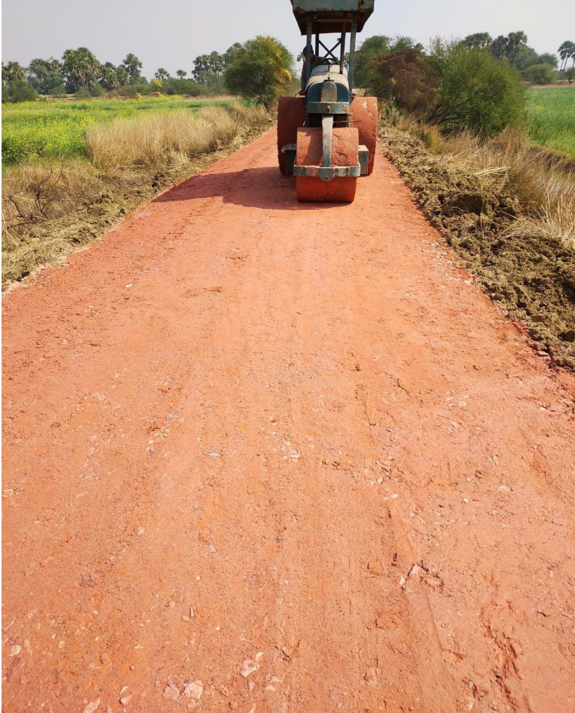
Figure 3.14 Rolling of binding material
