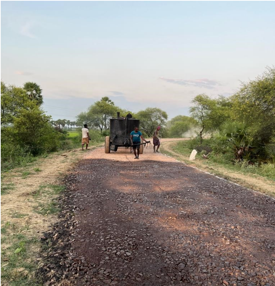
Figure 4.3 Spraying of bitumen emulsion using sprayer
