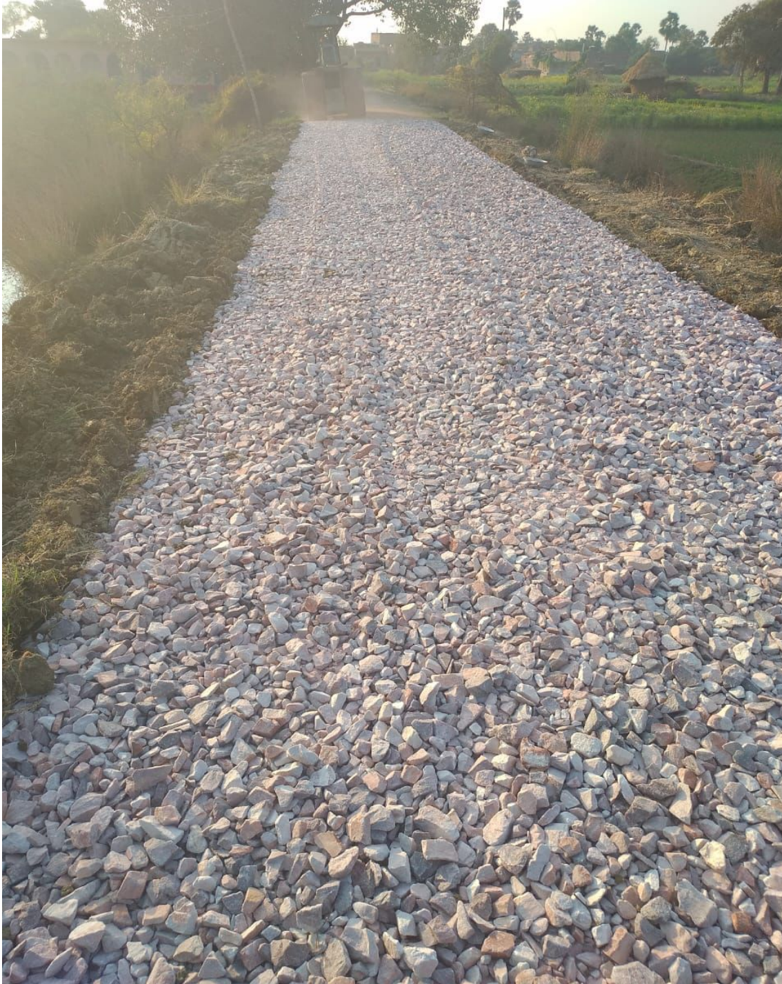
Figure 3.10 Rolling of WBM/ Grade-3
