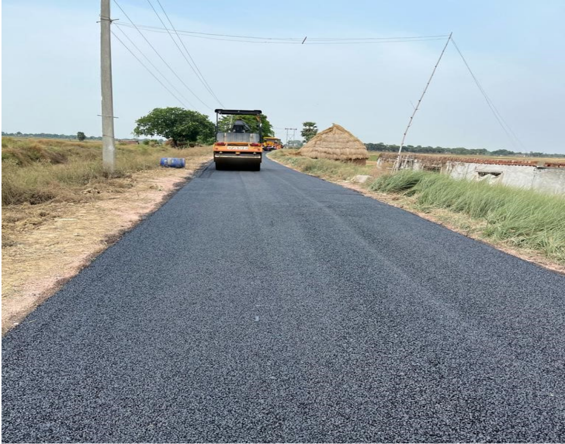
Figure 4.1 Laying and Rolling of SDBC
