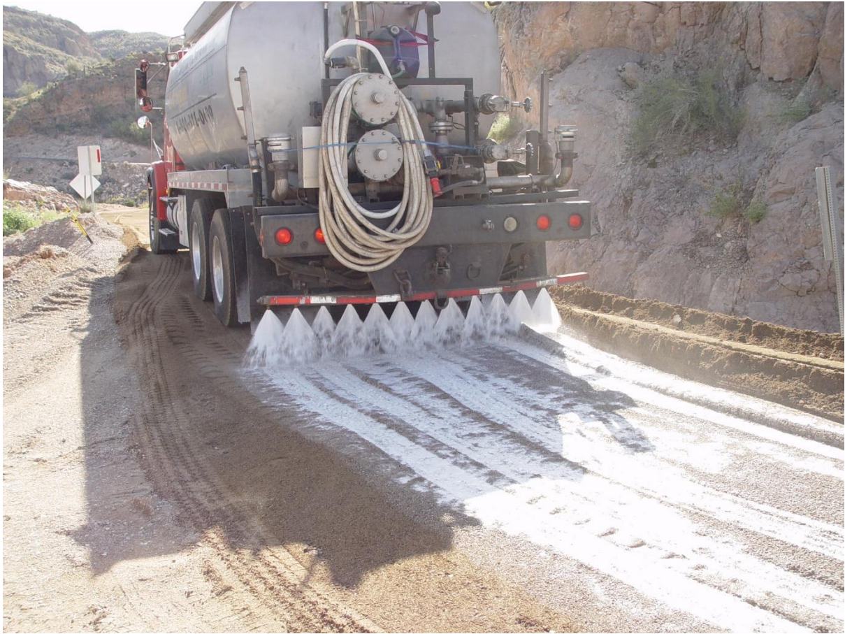
Figure 1.2 Chemical soil stabilization
