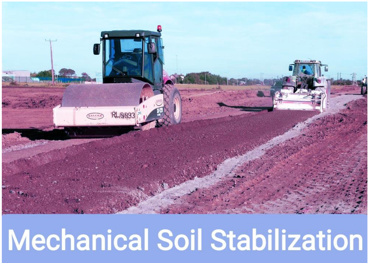
Figure 1.1 Mechanical Soil Stabilization
