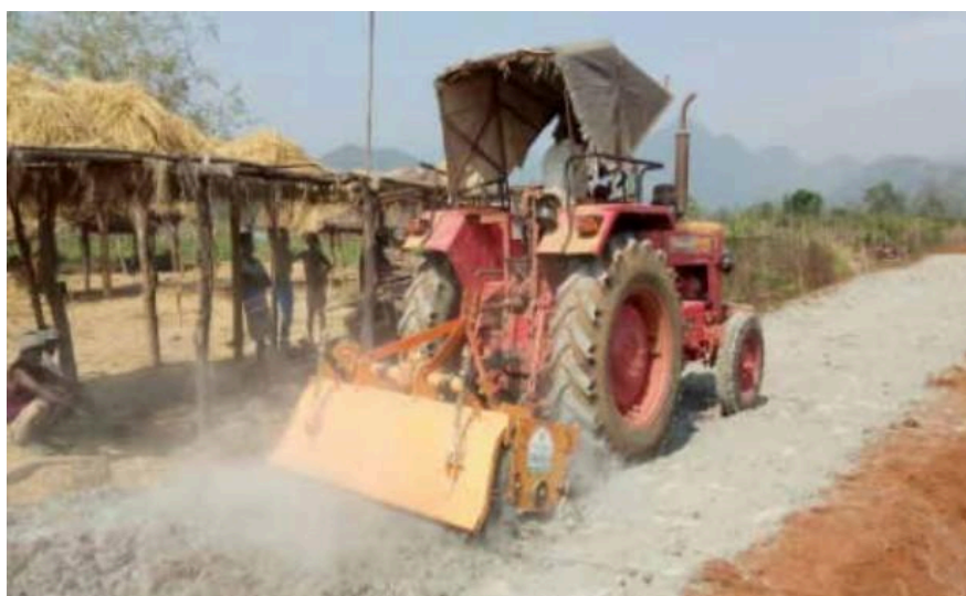
Figure 1.8 Cement Stabilisation
