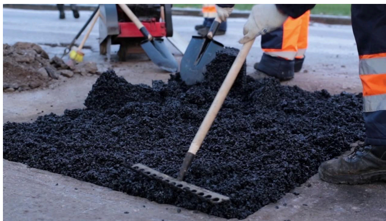
Figure 1.7 Laying of Cold Mix
