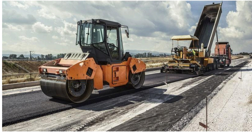
Figure 1.4 Laying of New Layer
