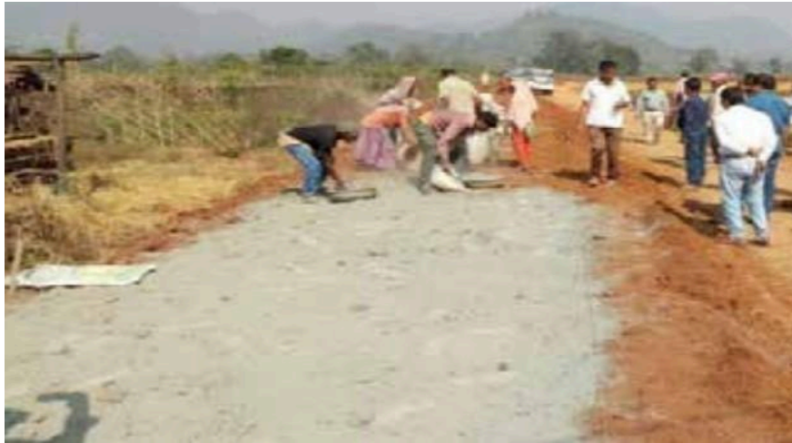
Figure 1.9 Cement Stabilizing
