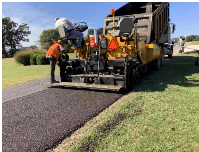
Figure 1.6 Laying of Cold Mix
