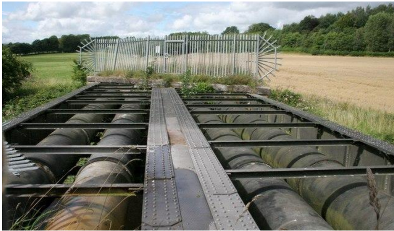
Fig. 1.1 - Four, 36-inch cast-iron pipes
