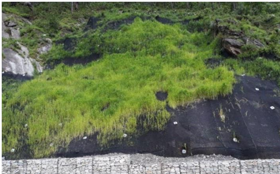
Figure 1.8 Vegetative cover on soft facing at Birahi, Uttarakhand
