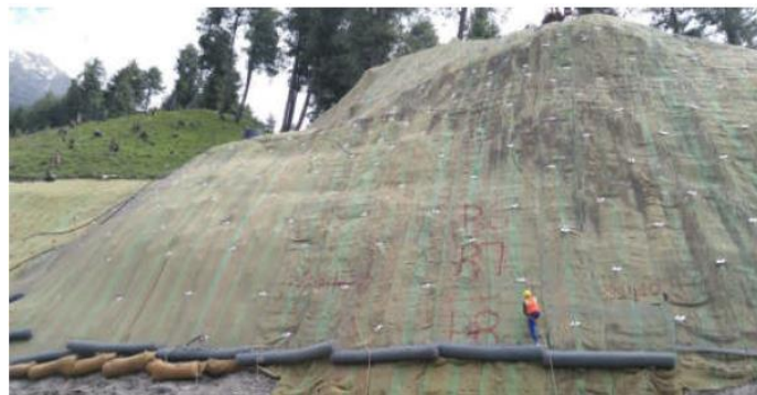
Figure 1.6 Flexible high tensile wire mesh wall Installed at Z-Morh Tunnel, J&K, India
