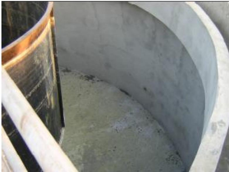
**Fig. 2.17:** Concreting Water Treatment Plant with Hyper 2000 (Source: R.N. Krishna [152])
