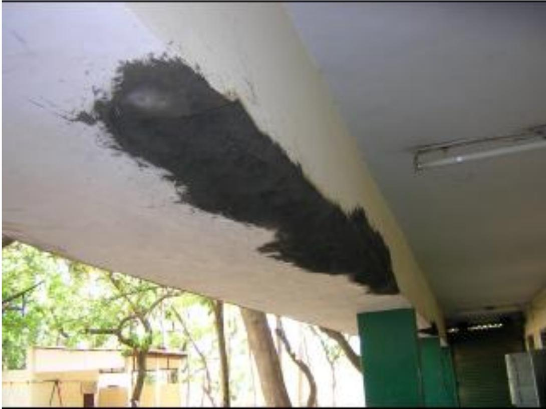
**Fig. 2.18:** Repair of RCC Beams with Hyper 2000 (Source: R.N. Krishna [152])
