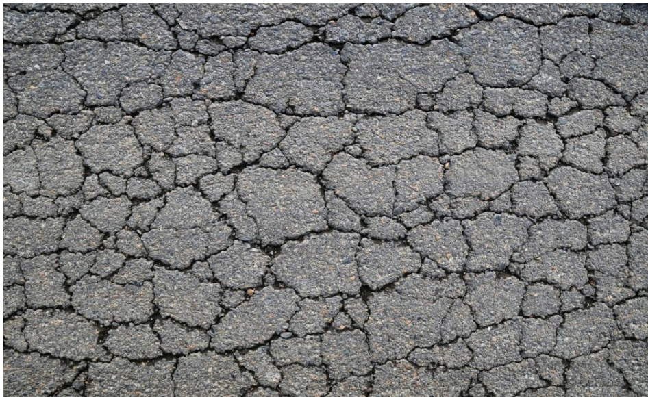
Figure 1.9 Alligator Cracking on Flexible Pavement
