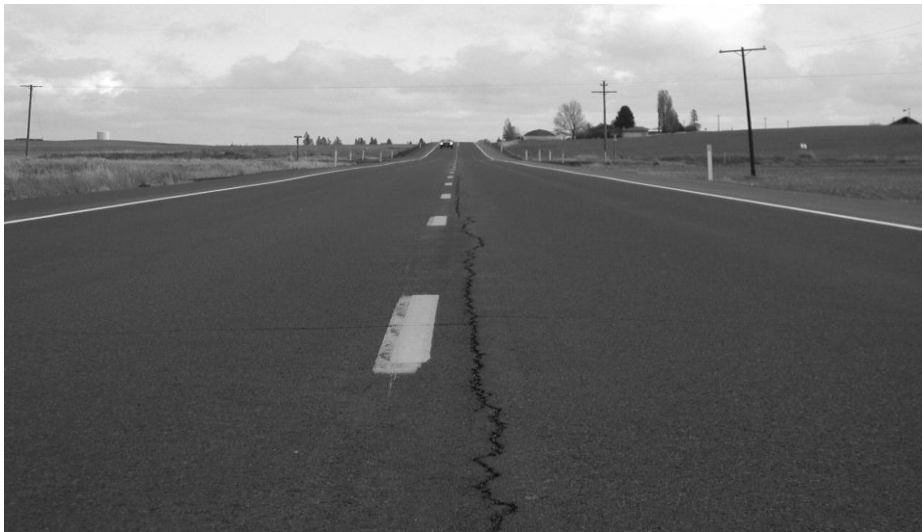
Figure 1.10 Longitudinal Cracking
