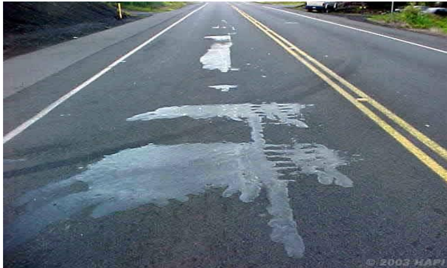
Figure 1.16 Bleeding on Pavement Surface
