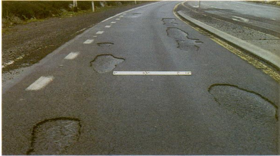
Figure 1.14 Delamination or Peeling of Asphalt Layer
