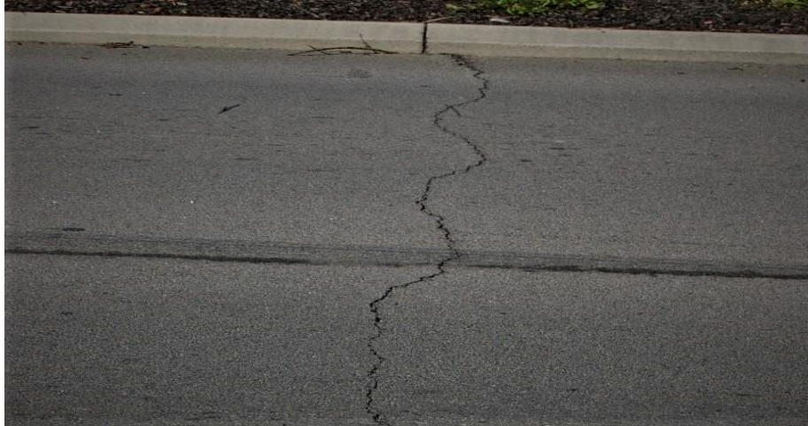
Figure 1.11 Transverse Cracking
