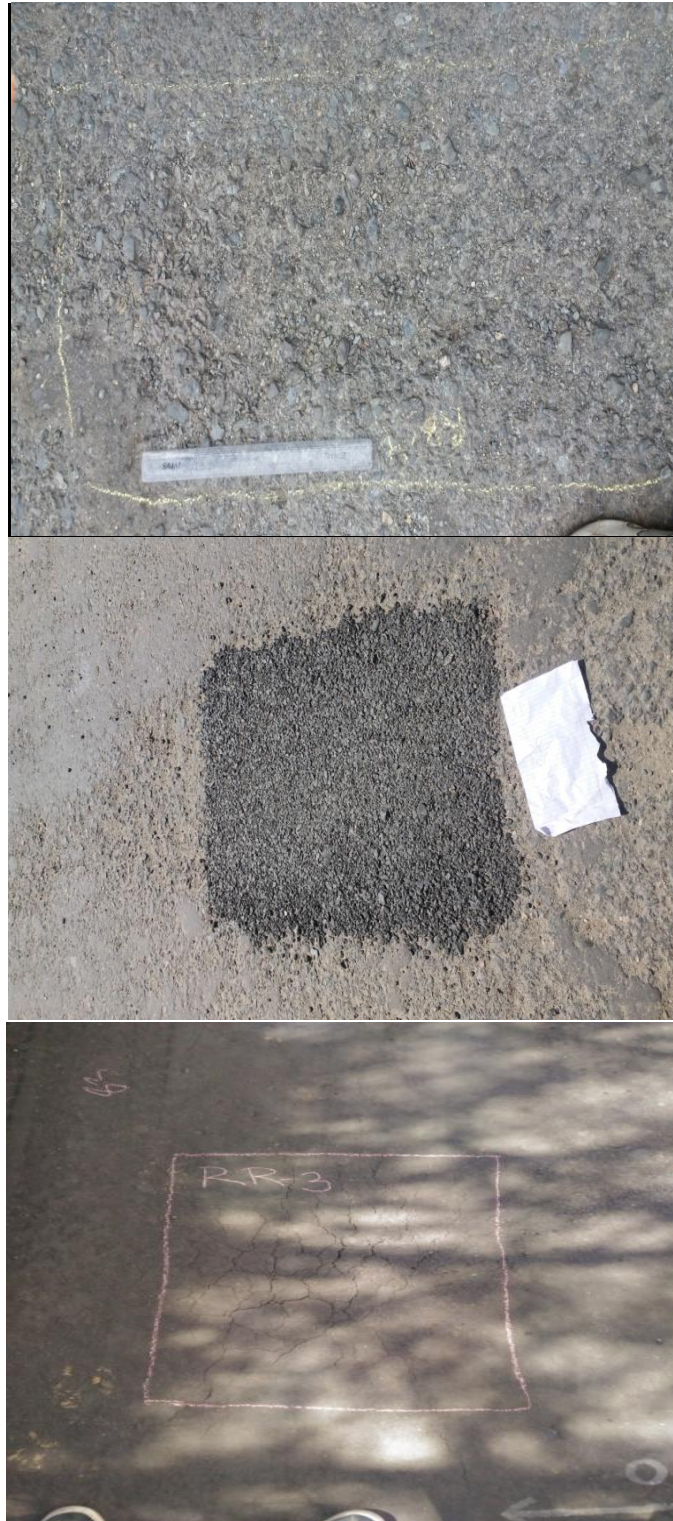
Figure 3.3 Measurement of Ravelling, Patching and Cracking on selected Rural Road Sections
