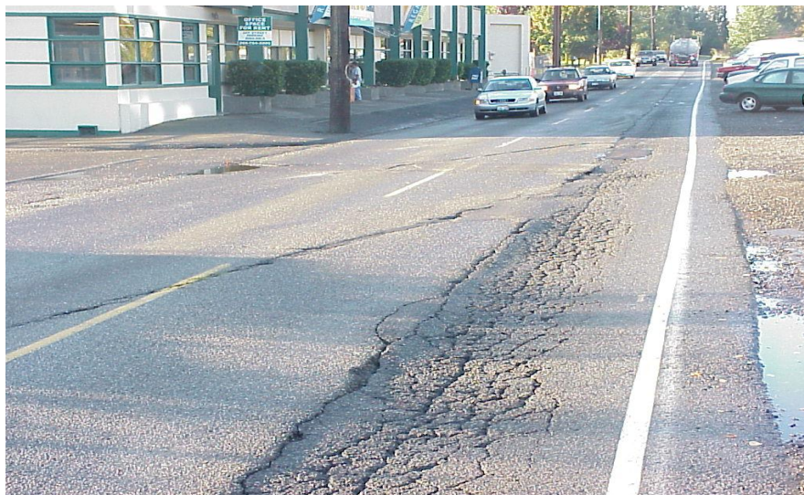
Figure 1.18 Rutted Surface of Bituminous Concrete Surface
