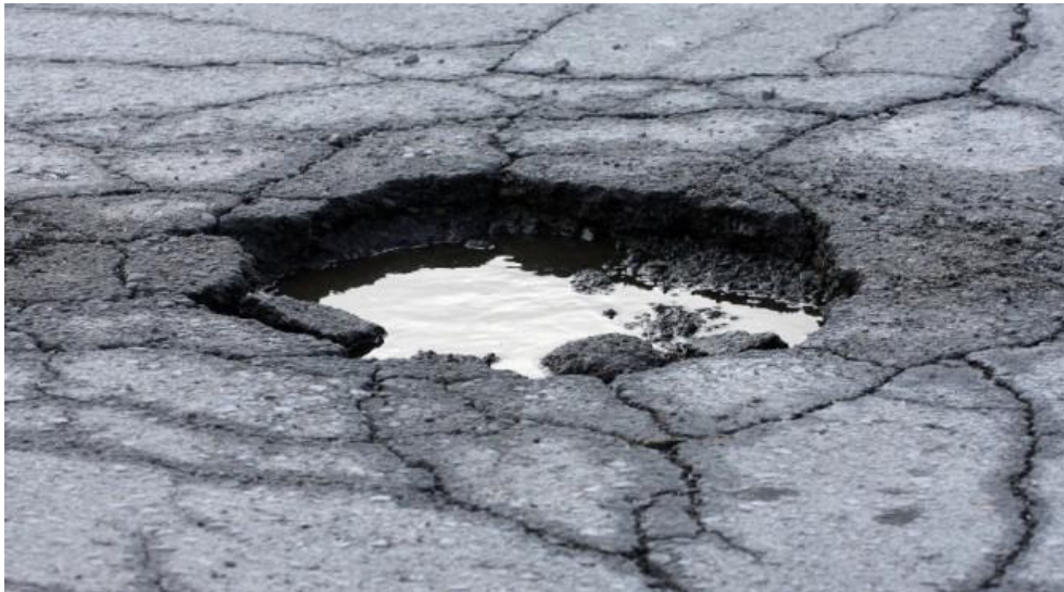
Figure 1.19 Potholes
