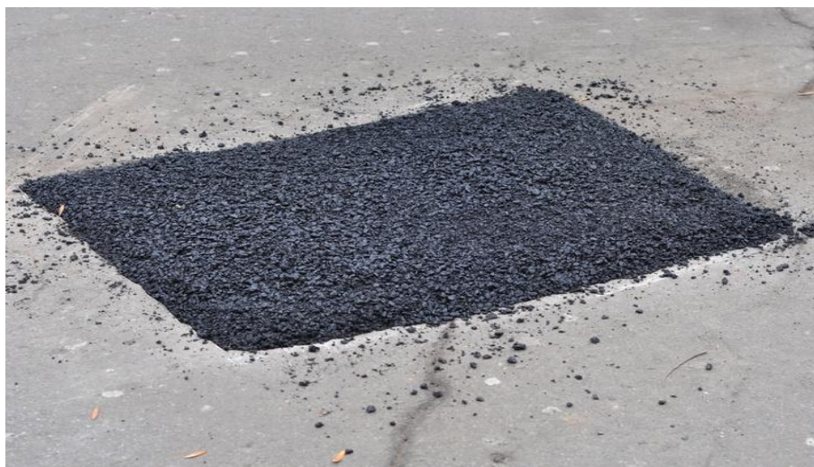
Figure 1.15 Patching of Pavement Surface
