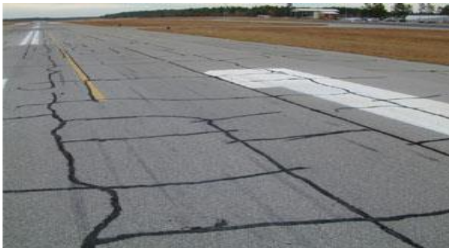
Figure 1.12 Block Cracking on Flexible Pavements
