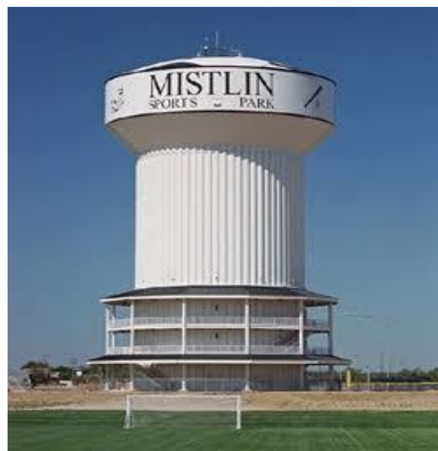
Figure 10: Front view of Fluted pillar water tank
