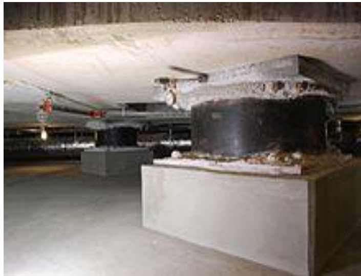
Figure 13: Base isolators under the Utah state capitol
