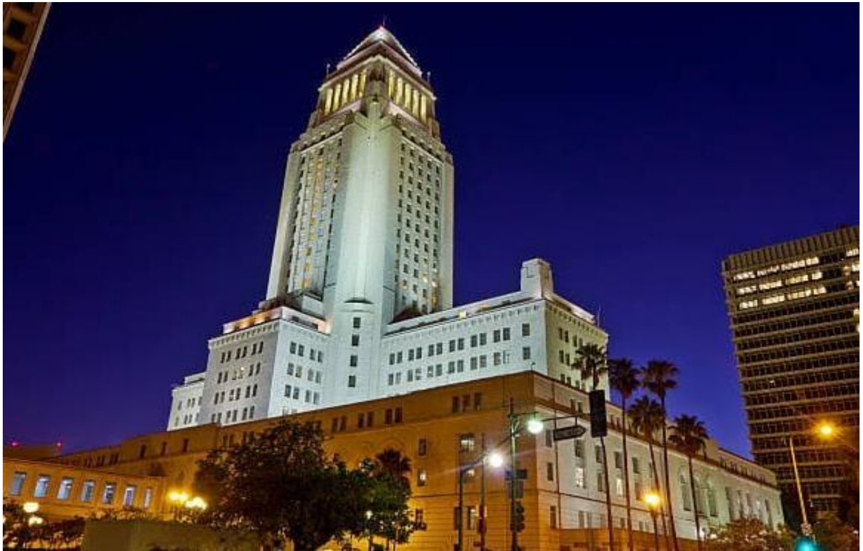
Figure 12: LA city hall retrofitted with base isolation
