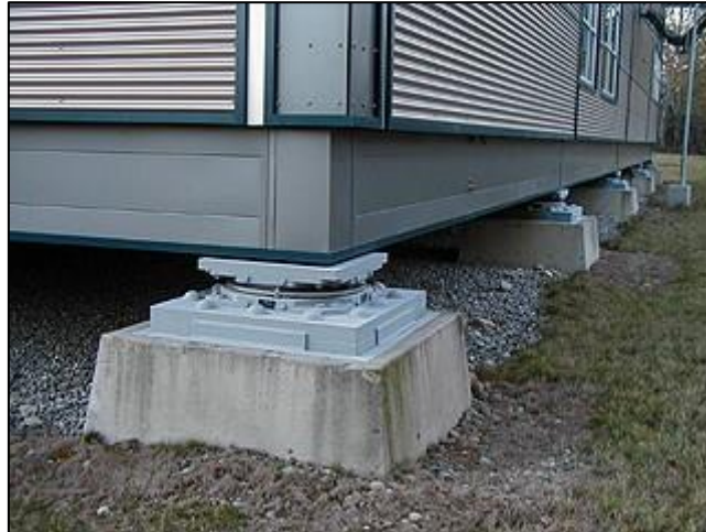
Fig. 17 Sliding Isolator
