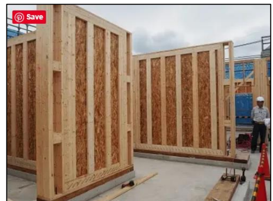
Fig. 28 MIDPLY Shear Wall
