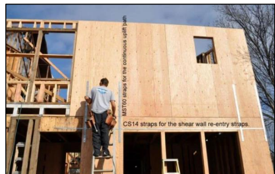
Fig. 27 Plywood Shear Wall
