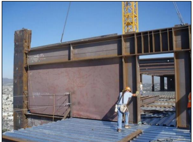
Fig. 30 Steel Plate Shear Wall
