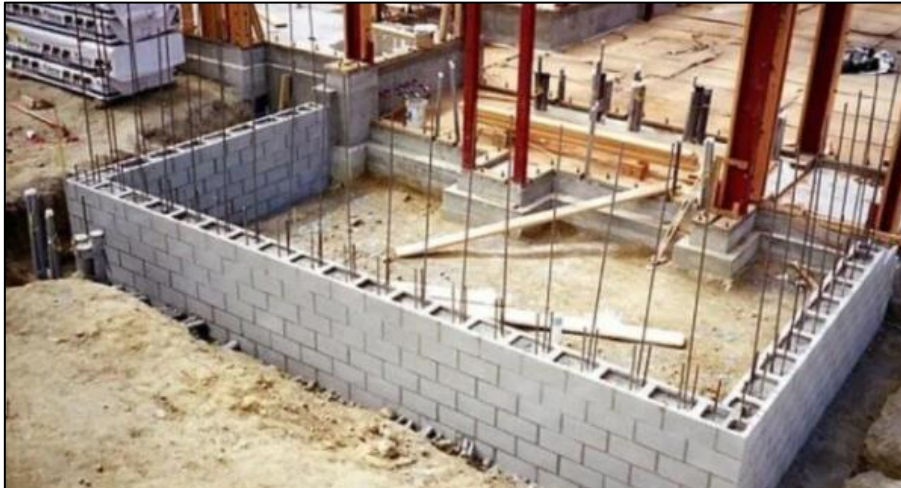
Fig. 29 RC Hollow Concrete Block Shear Wall
