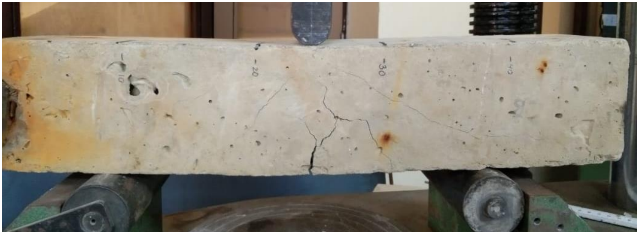
Figure 4.6 Experimental Crack pattern of Corroded Beam
