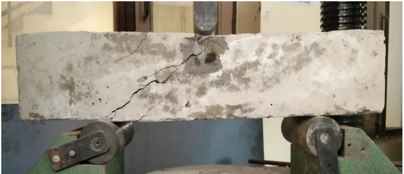
Figure 4.2 Experimental Crack Pattern of Control beam.
