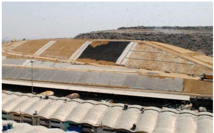
Figure 1. 7 Geocell mat laid over the slope which helps in strengthening the soil and holding the top soil layer tightly. [2]
