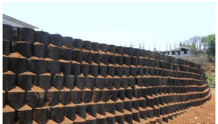
Figure 1. 9 Geocells used to stabilize retaining wall. [2]
