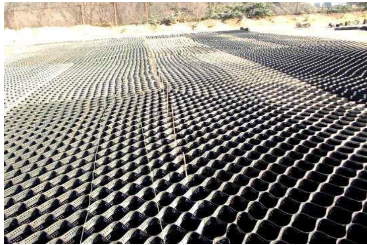
Figure 1. 8 Geocells laid for soil stabilization. [2]
