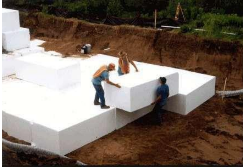
Figure 1. 6 EPS geofoam in cubical form is the extruded polystyrene large lightweight blocks easy to handle and apply[4]
