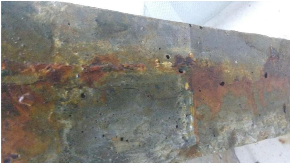
Figure 4.22 - Cracking propagation due to corrosion
