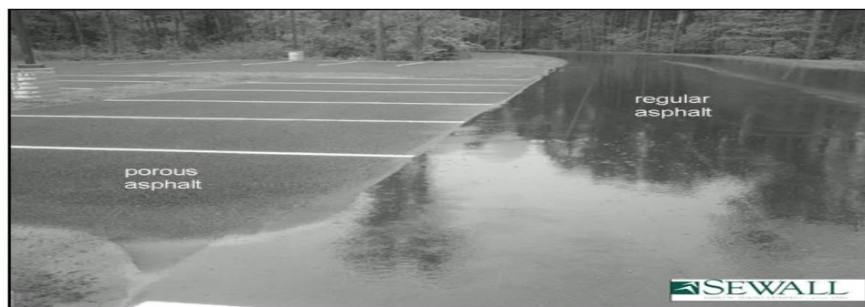
Figure 2.5:- Permeable Pavement Vs Normal Asphalts
