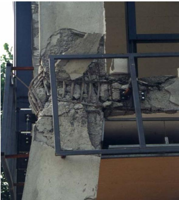
Fig. 2.3.2 Loss of grip at joint region
