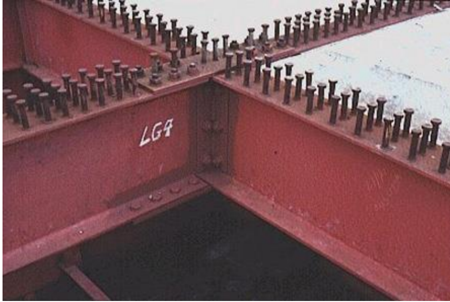
Figure 3.b Composite Beam
