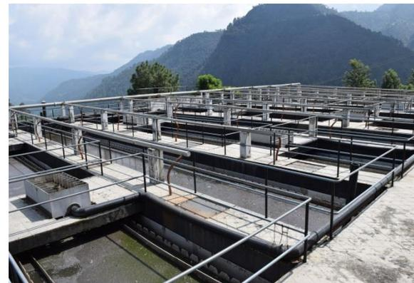
**Plate 1.6:** UASB Reactor
