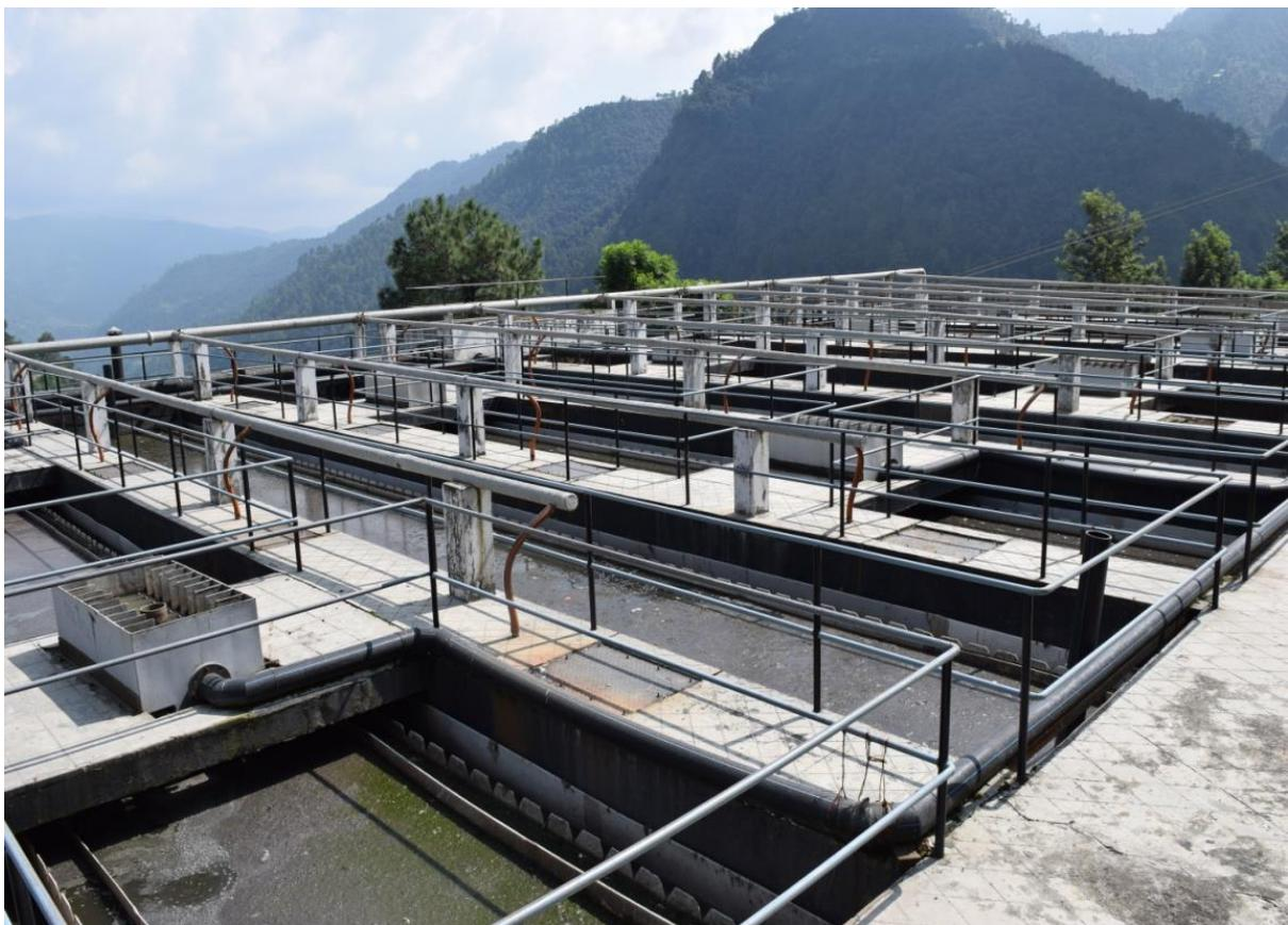
**Plate 1.9:** Full Scale UASBR located in Lalpani STP
