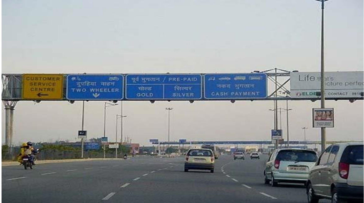
Figure 4: Delhi Noida Toll Bridge
