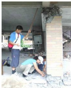
Measuring of column drift
