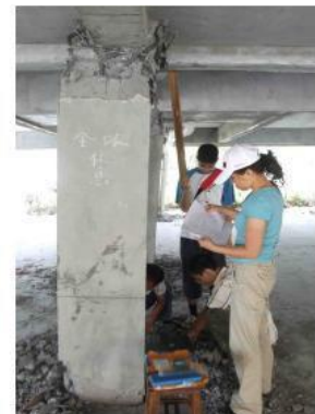
Joint damage
