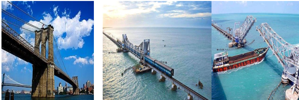
Figure 1.4: Brooklyn Bridge, USA and Pamban Bridge, India
