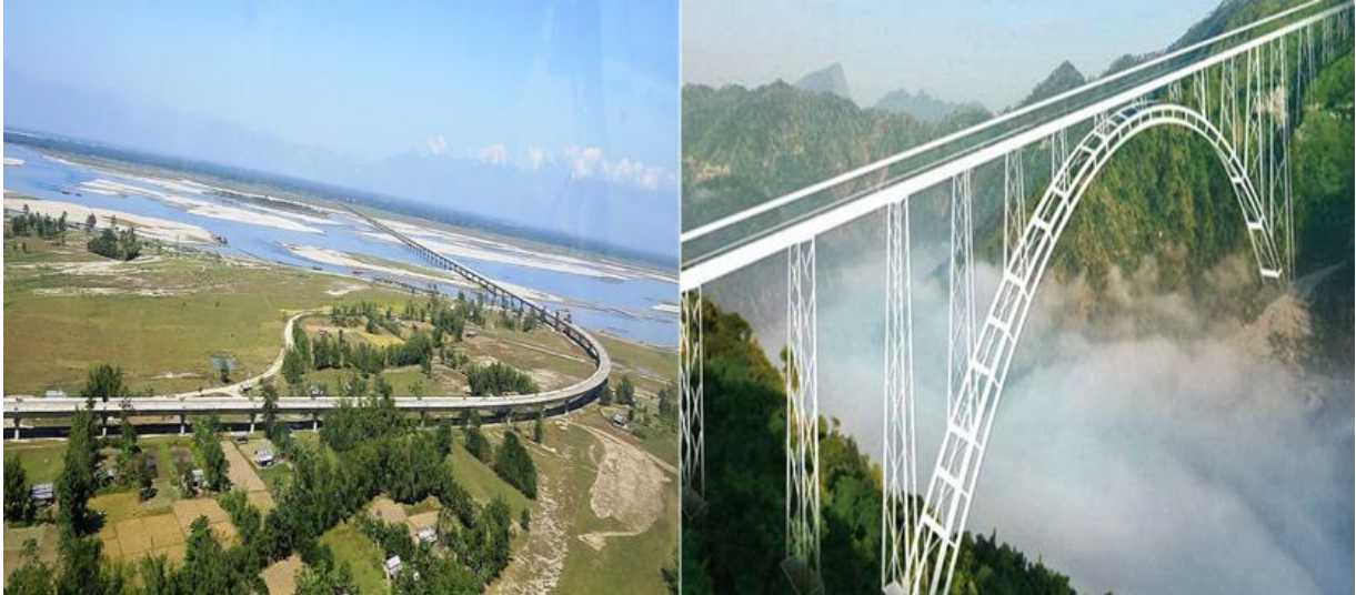
Figure 1.1: Dhola-Sadiya Bridge (Beam Bridge) and Chenab Bridge (Rail Bridge)
