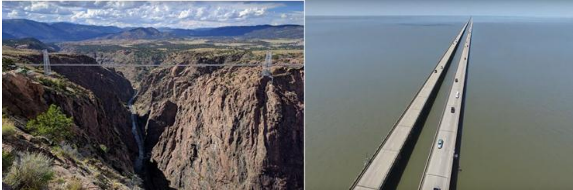
Figure 1.2: Royal Gorge Bridge (Suspension Bridge), USA and Lake Ponchartrain causeway Bridge, USA
