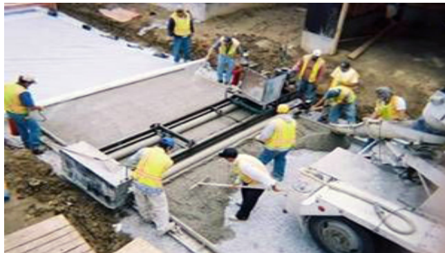
Fig.1.1. Laying of fresh concrete (source: Md. Aminur Rahman et al. [11] ).
