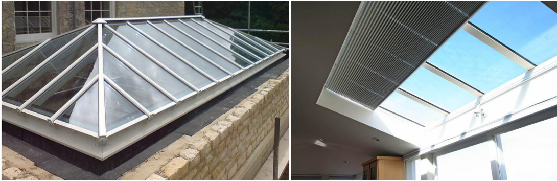
Fig – 4.10 Sloped Glazed Roof
