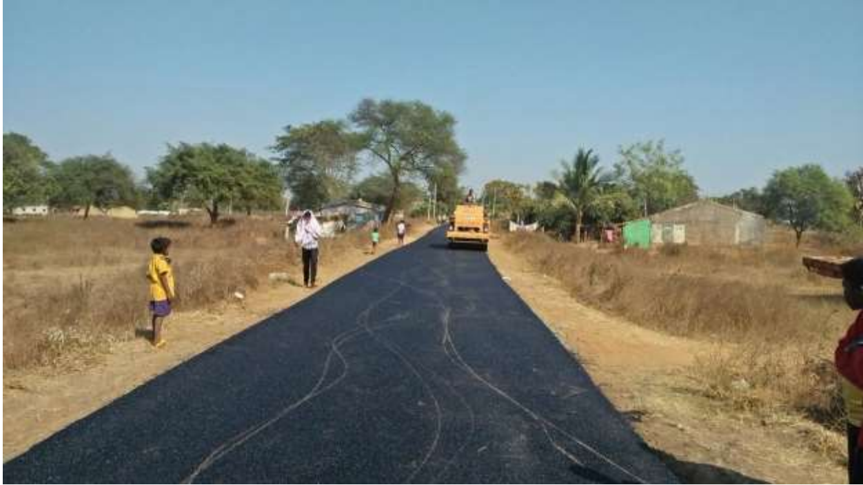
Fig 1.1 Construction of SDBC pavement
