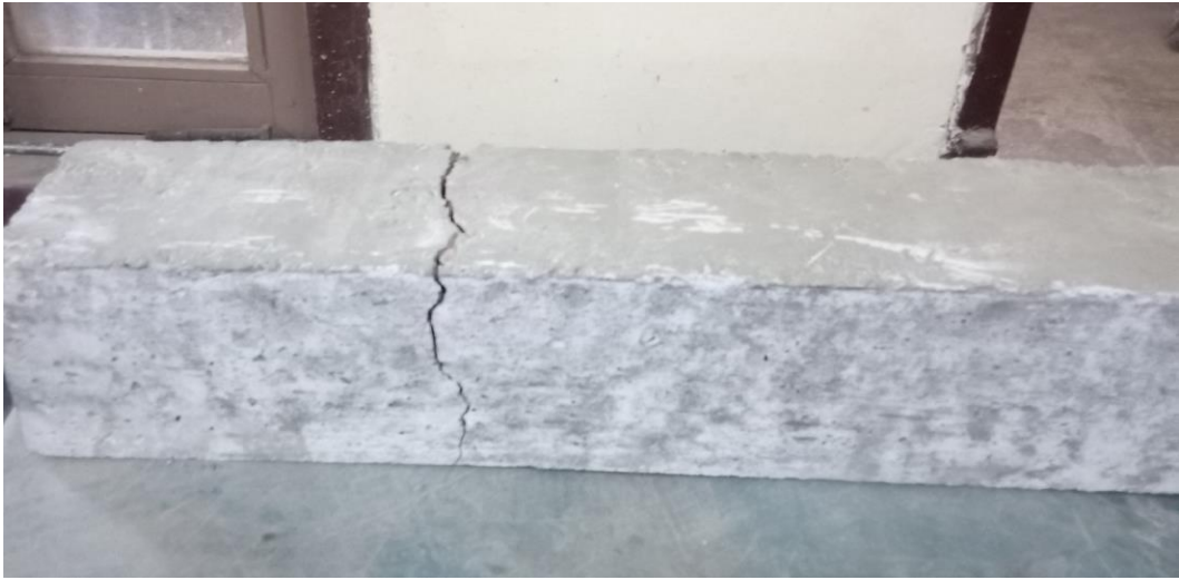
Figure 4.6 Beam Failures under FTM
