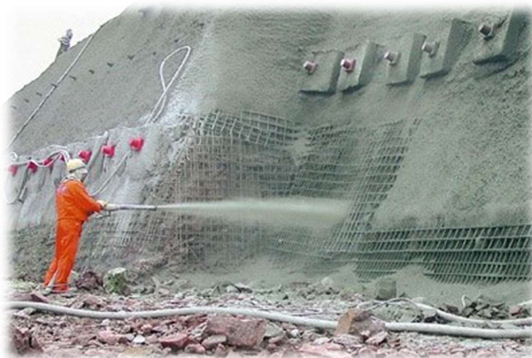
Fig 1.3: Shotcreting is done with the help of a pipe with a nozzle
