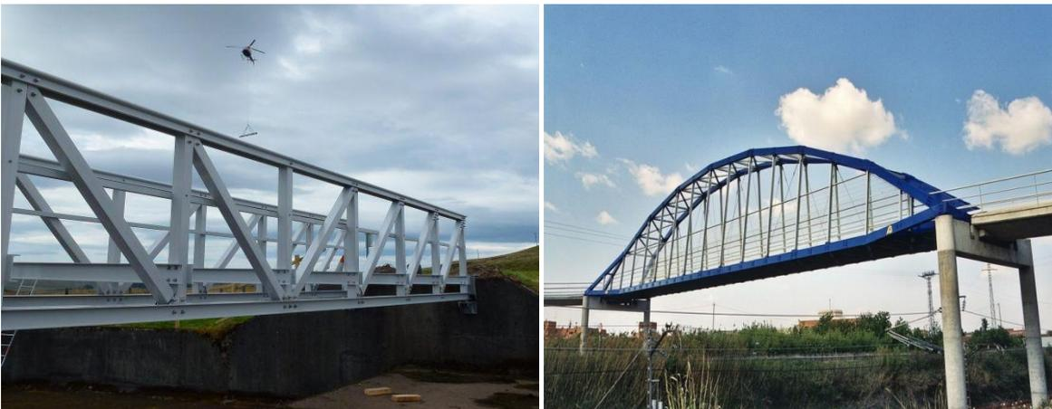
**Figure 1.6** Bridges made of FRP
