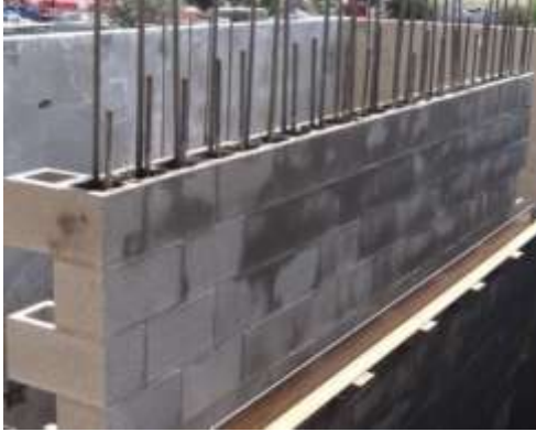
Reinforced masonry shear wall
