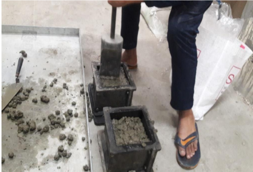
Fig 3.14 Tampering of cube
