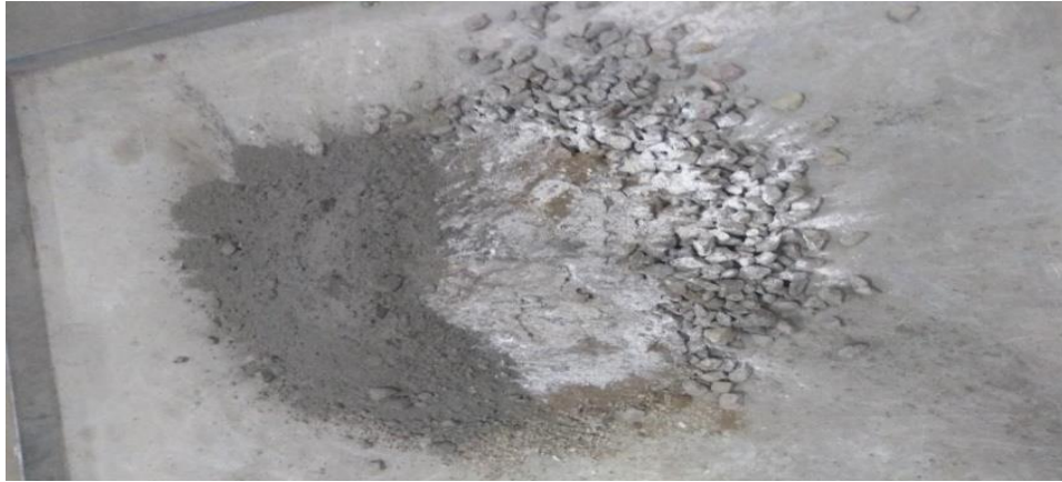
Fig 3.12 Mixing Of Concrete
