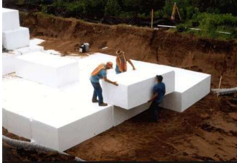
Fig. 1.6 EPS geofoam in cubical form is the extruded polystyrene large lightweight blocks easy to handle and apply[12].
