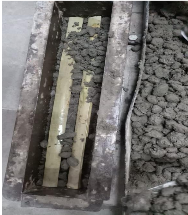
Figure 3.15 (a) Bamboo as Reinforcement
