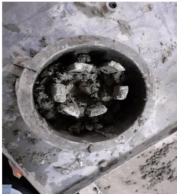
Figure 3.20 Sikadur 32-Gel coated Reinforcement
