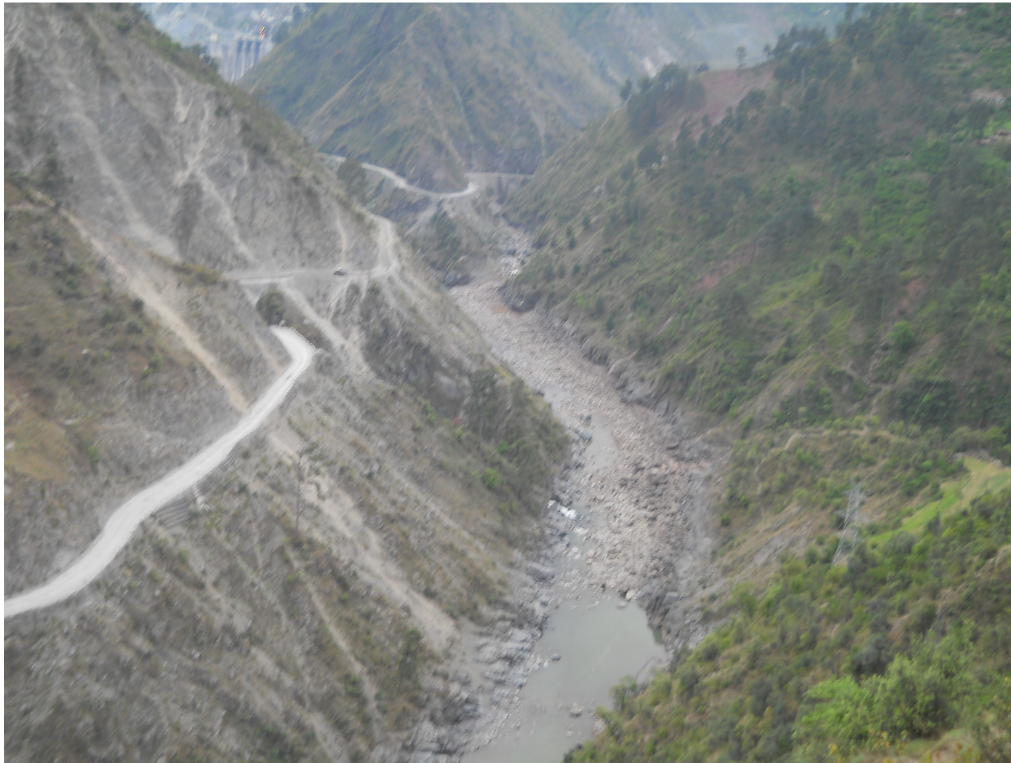
Figure-4.9: D/s View of River and Dam
