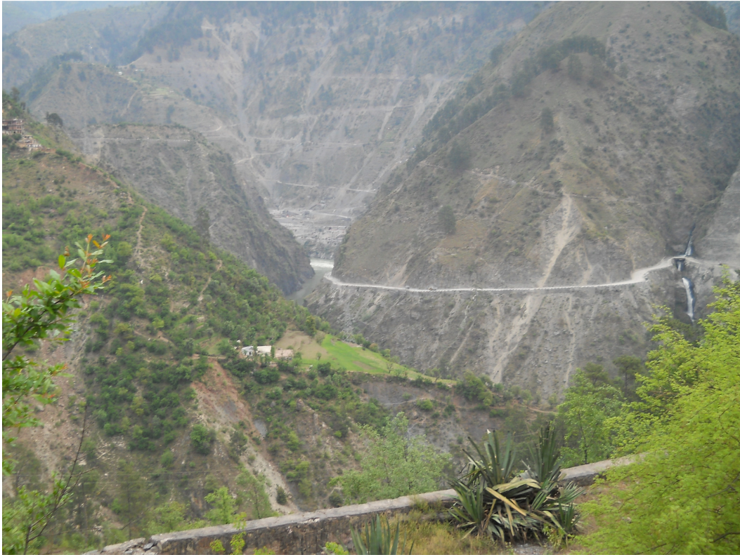
Figure-4.7: View of TRT outlet fall and Gajpat Nala
