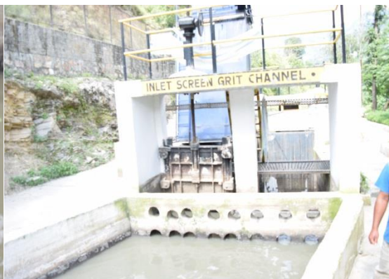
Figure 1.3: Screen Channel
