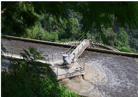
Figure 1.6: Aeration Tank
