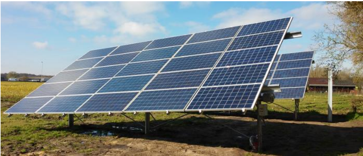
Fig 2.1: single axis solar tracking system
