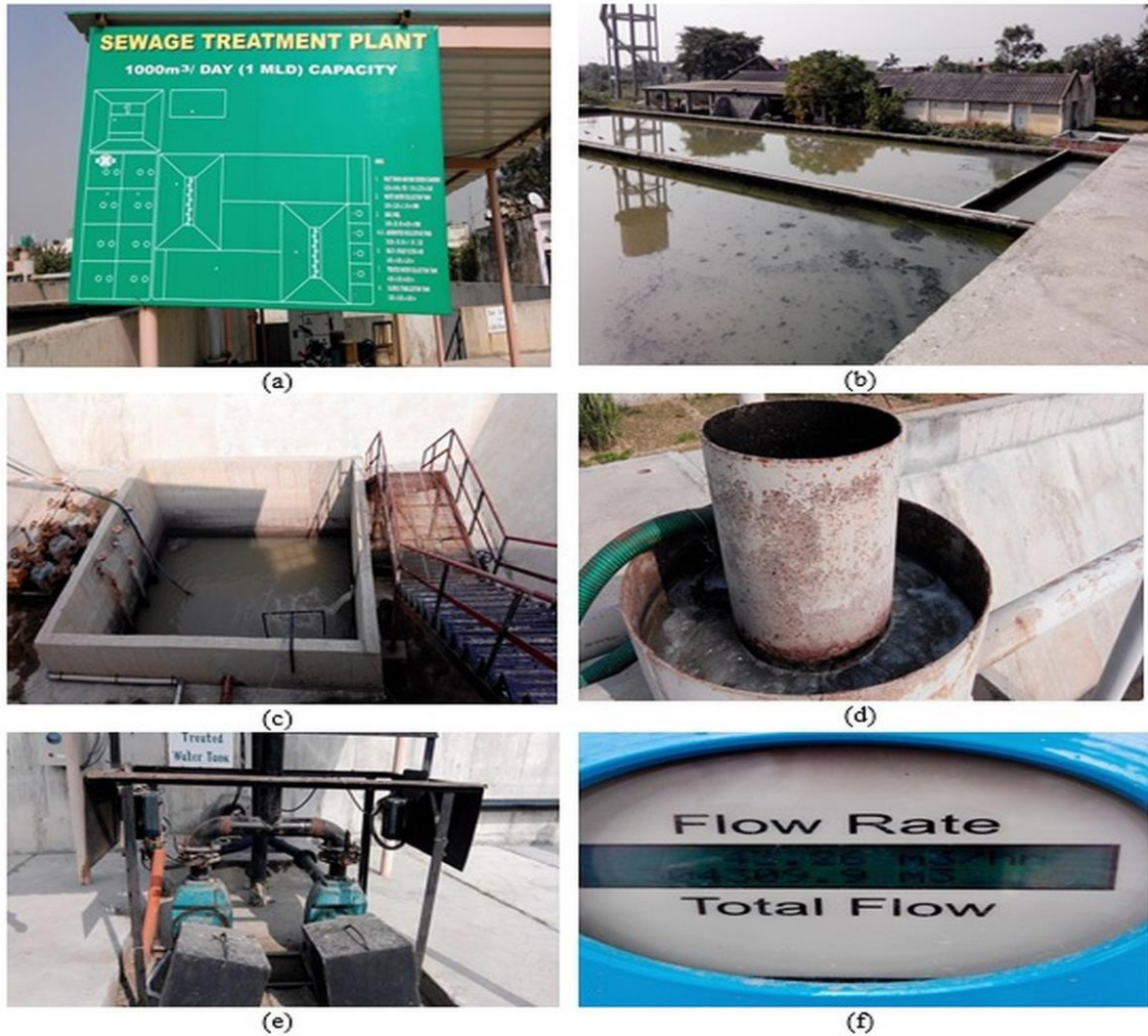
Figure 3.4: Site location: sewage treatment plant (a) model of sewage treatment plant, (b) augmented facultative pond, (c) wastewater collection tank, (d) bar pipe, (e) motor for treatment of water and (f) total flow rate of treated water
