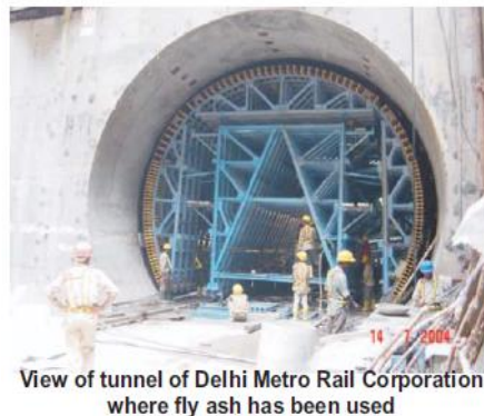
Fig. 1.3: A Delhi Metro Tunnel Where Fly Ash Has Been Used.
