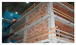
Fig. 4: Adding infill wall
