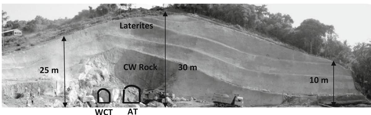
**Fig. 2** Pictorial view of the portal area during construction. AT access tunnel, WCT, water curtain tunnel, CW completely weathered
