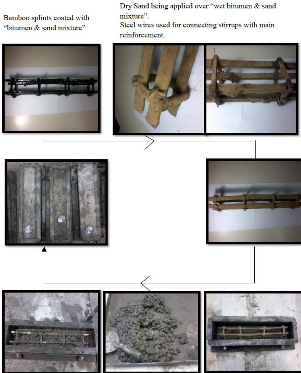
Figure 3: Preparation of MBRCC beam elements (Type - III).
