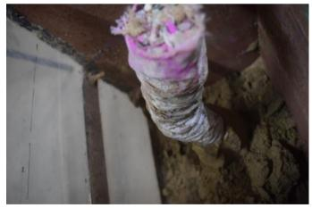
(c). Vertical reinforcement column failure due to bulging
