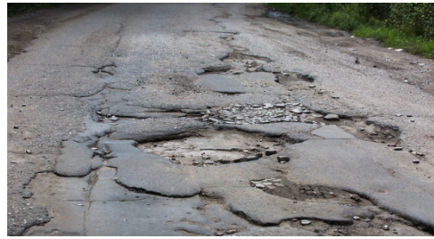
Figure 1.1 A pothole
