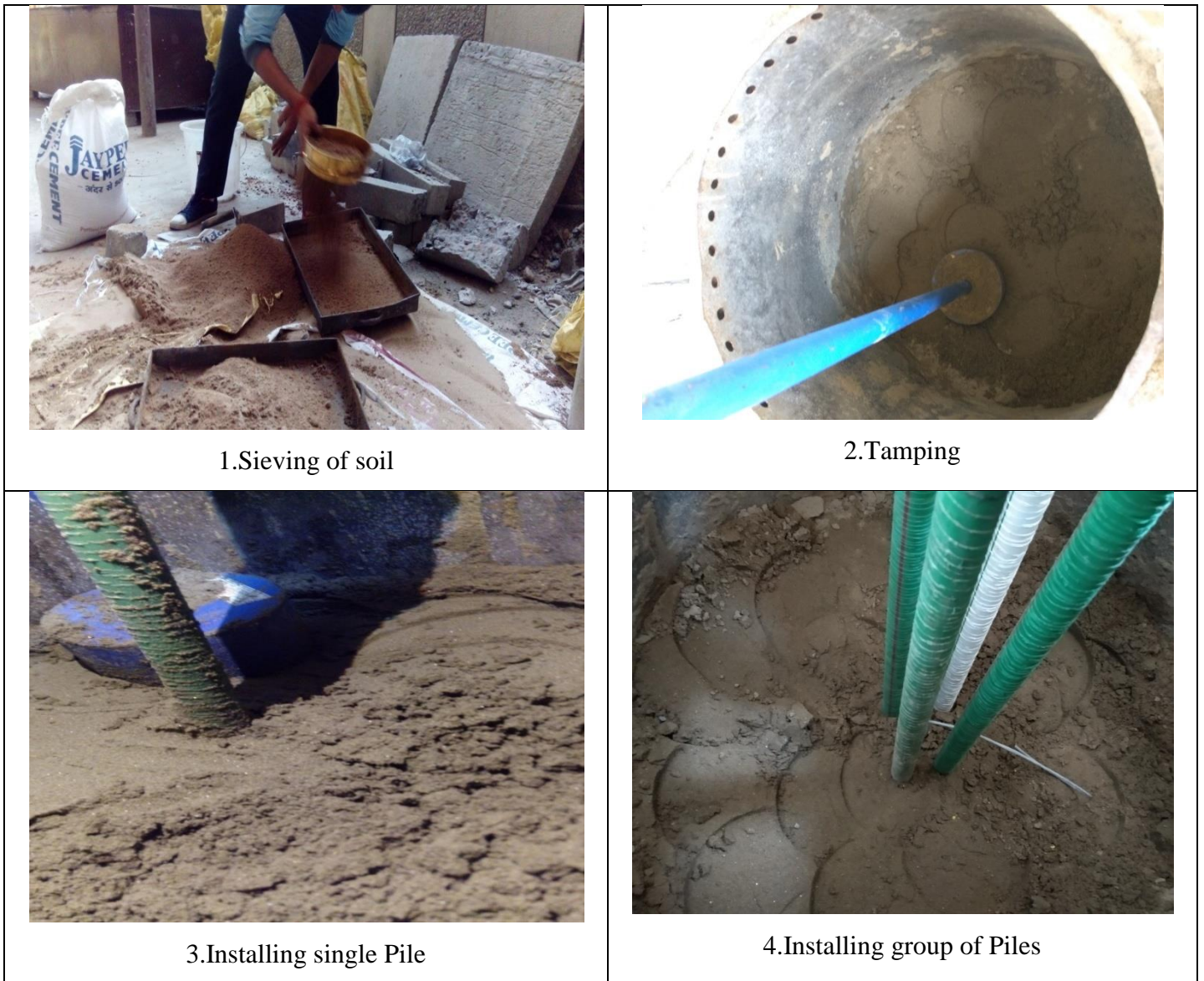
Figure 3.15 - Installation of pile
