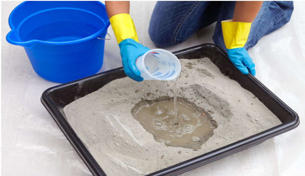
Fig 7: water added to concrete
