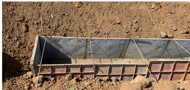
Figure 3.4.2 (B) Head wall of pipe culvert
