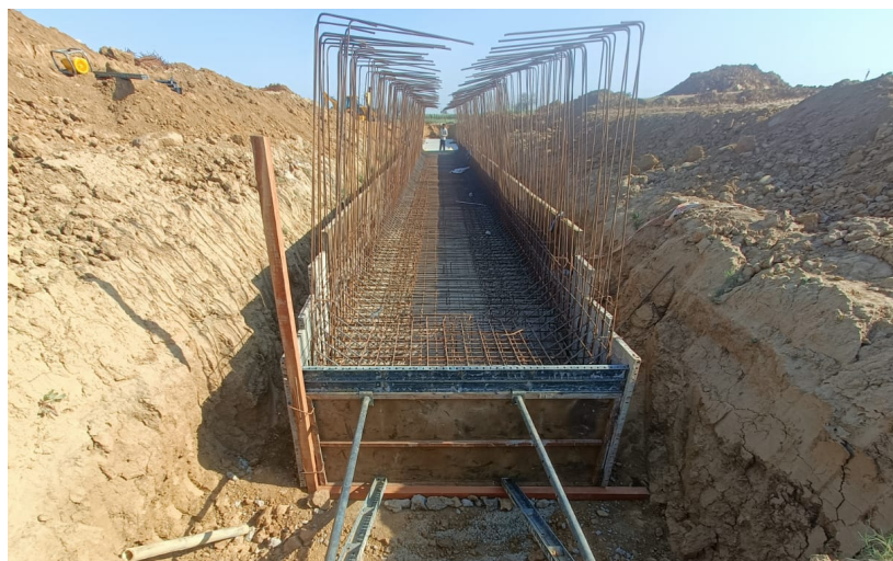
Figure 3.3.2 Structure ready for concreting (3.5 x 3.5m) (A)
