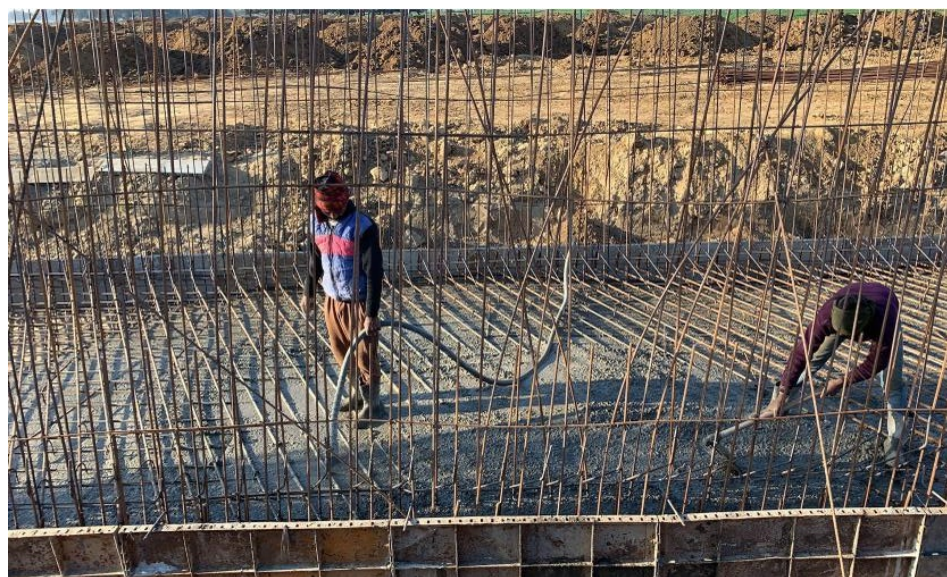
Figure 3.2.3 Concreting of Rafting (Total concrete used = 33 cum.s)
