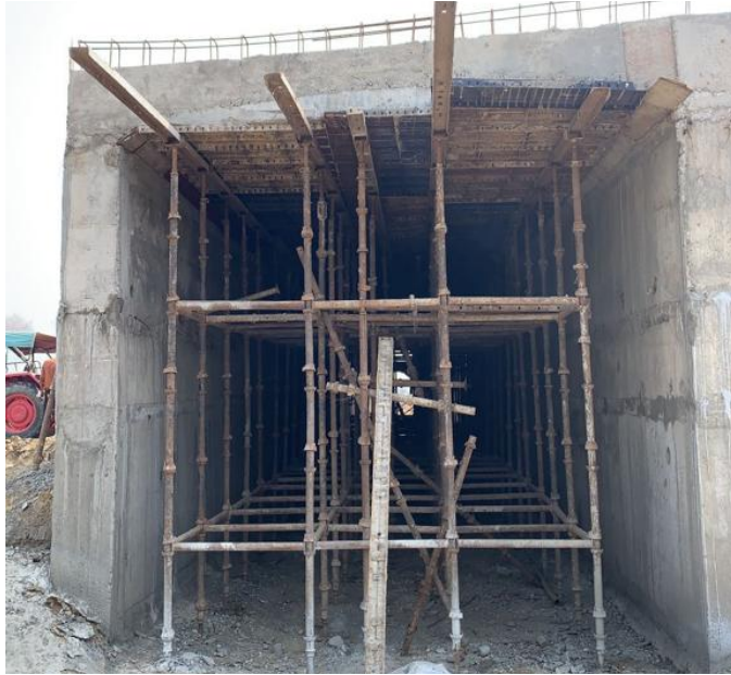
Figure 3.3.2 Structure completed, removing of staging left (B)
