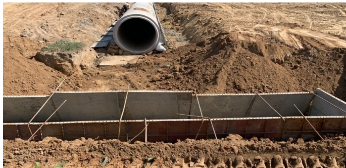
Figure 3.4.2 (A) Head wall of pipe culvert
