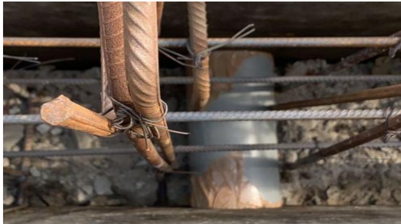
Figure 3.2.4 (A) Weep hole at Side wall
