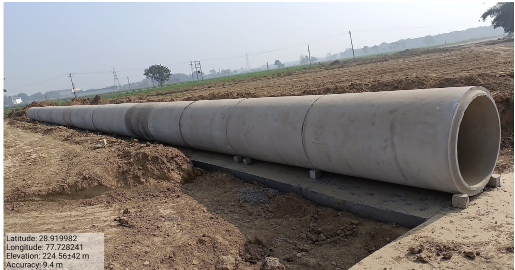
Figure 3.4.2 Laying of Pipe Culvert
