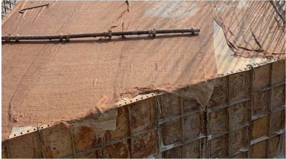
Figure 3.1.6 Curing of Slab and wall
