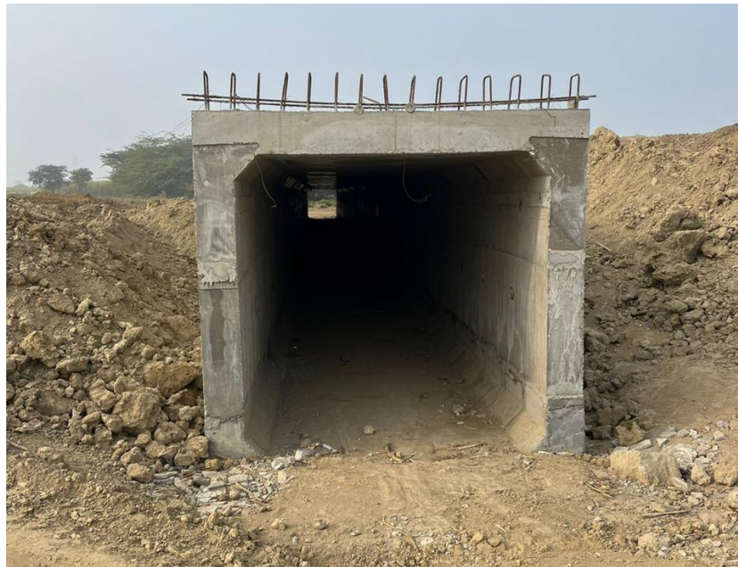
Figure 3.3.2 Box culvert at 13+600 (C)
