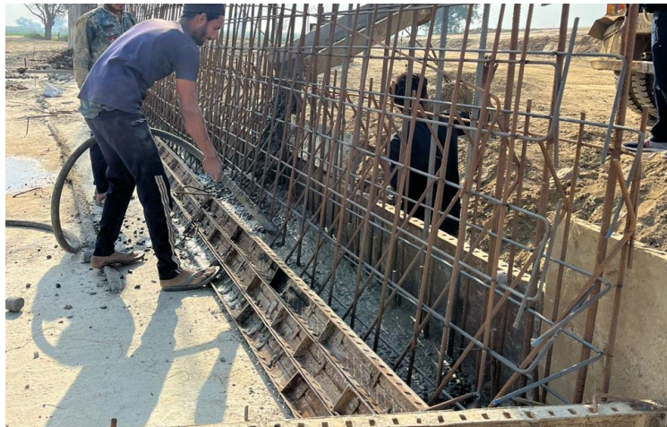
Figure 3.1.5 Concreting of Haunch (250X250mm)
