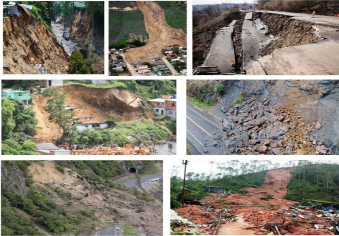
Fig 2.5 landslide in hilly areas
